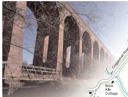
Chappel Viaduct, Chappel
